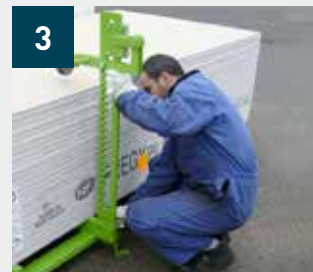
Adjustable retaining arms fitted
